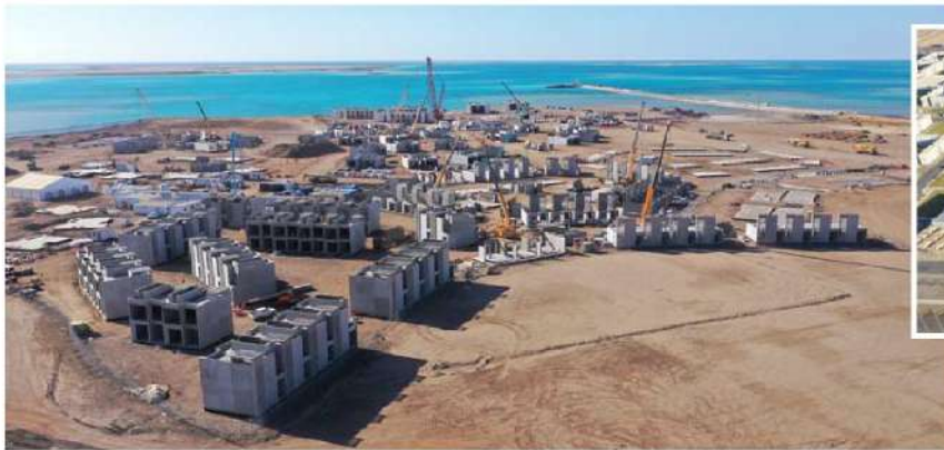
Work in progress on the Coastal Village.
